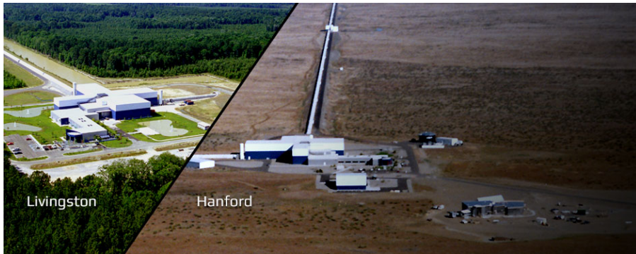
Figure 1.3. The Advanced LIGO system in Livingston, USA (left), detected the first gravitational wave, which was subsequently, about seven-thousandths of a second later, confirmed by the Advanced LIGO system in Hanford, USA (right) (figure reprinted from https://www.ligo.caltech.edu ).
