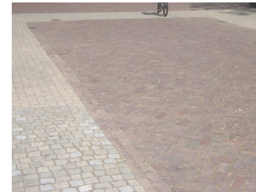
central strip in Dutch clinkers flanking strips in concrete bricks
