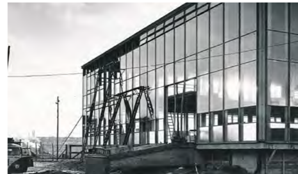
E-hal (Impuls) under construction approx. 1959.
