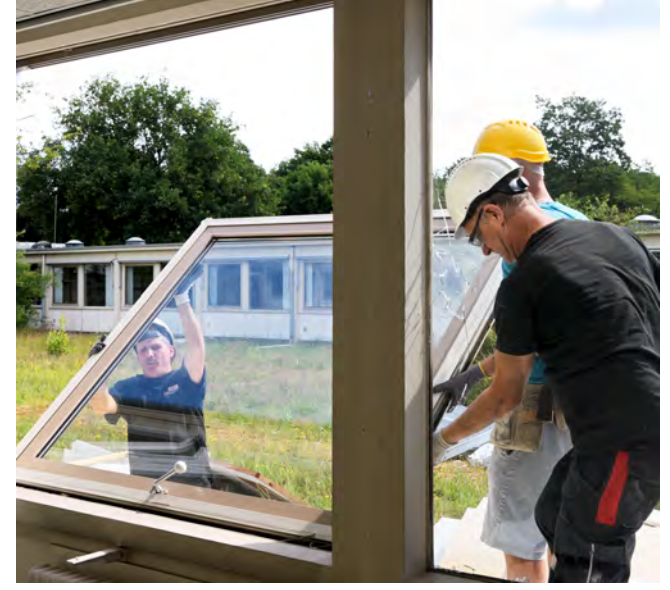
Photo: Dismantling of the pavilion's windows, which are reused at Skatehal Area 51 in Eindhoven. (Photo Bart van Overbeeke)
