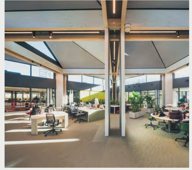
Photo: In Neuron, a wooden structure was chosen in the atrium, which stores CO 2 . Sustainable materials and vintage furniture parts were also selected for the furniture. (Photo Jannes Linders)
