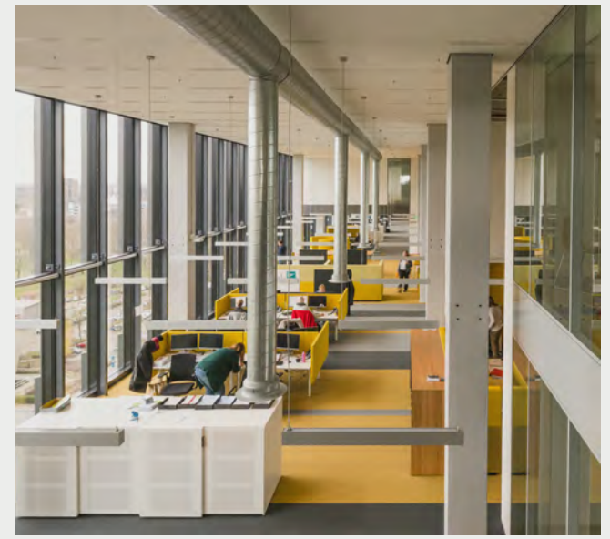
Photo: In Atlas, the built-in flexibility of the original design was well utilized during the renovation: every odd-numbered floor has a steel structure that is easy to remove, allowing for the creation of large open spaces that promote connection. (Photo Jannes Linders)
